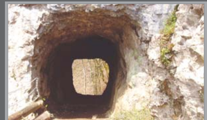
THE AKERRETA TUNNEL
